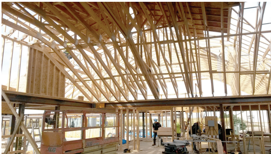
The steel beam framework required clear spans of 50-62 feet.
