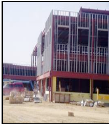
Non-load bearing exterior wall framing
