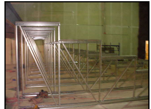
Frames for stadium seating installed.
