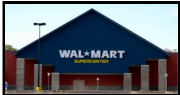
Exterior view of the completed main entrance.
