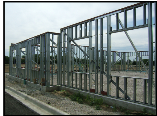
Wall panels used as bearing walls.
