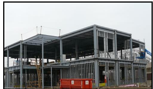
Wall panels used as non-load bearing walls.
