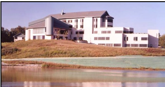
Exterior view of the monastery with the four-acre lake which provides geothermal heating and cooling.
