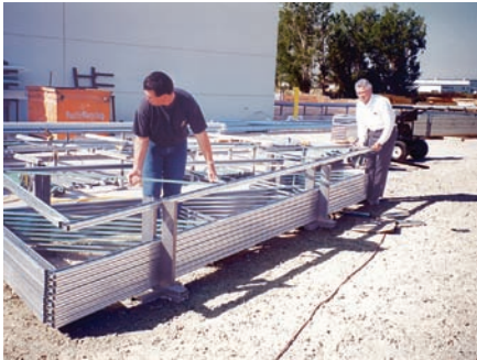
TrusSteel trusses are often light enough for two men to unstack and stage.
