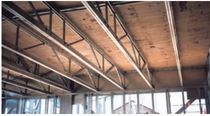
TrusSteel floor trusses provide the convenience of open web members.
