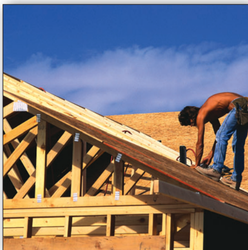
Permanent bracing system
