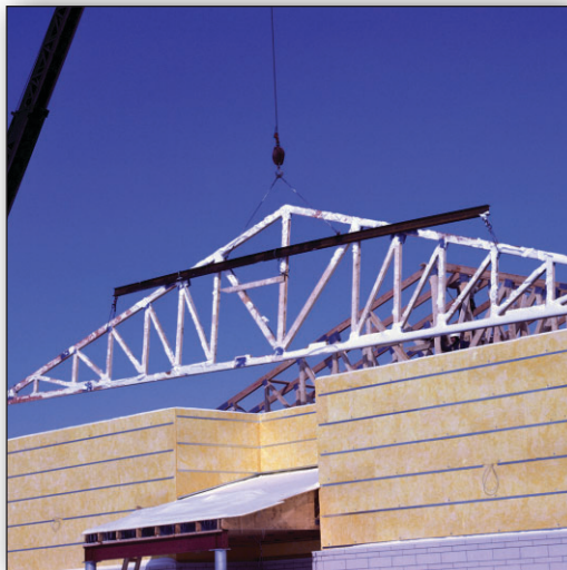
Erecting the trusses on the jobsite
